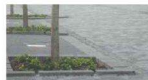
FIGURE 19.16: EXAMPLE OF INLETS TO ALLOW SURFACE WATER RUNOFF TO INFILTRATE INTO TREE PITS. TAKEN FROM CIRIA REPORT C753 THE SUDS MANUAL.
