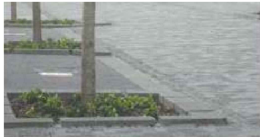
FIGURE 19.16: EXAMPLE OF INLETS TO ALLOW SURFACE WATER RUNOFF TO INFILTRATE INTO TREE PITS. TAKEN FROM CIRIA REPORT C753 THE SUDS MANUAL.
