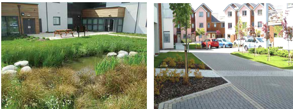
Figure 4-1: Images of a Rain Garden and Permeable Paving
